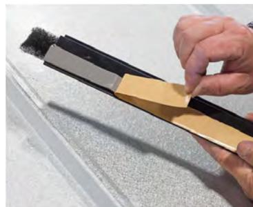
**STEP 2:** Peel away the backing from the butyl tape. Allow the over-stuffed foam to expand so it completely fills the gap between the top of the rib and the SSV. Align the SSV along the chalk line.
