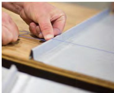
**STEP 1:** Snap a chalk line about one-eighth to one-sixteenth of an inch above the position where the ridge cap will be installed.
