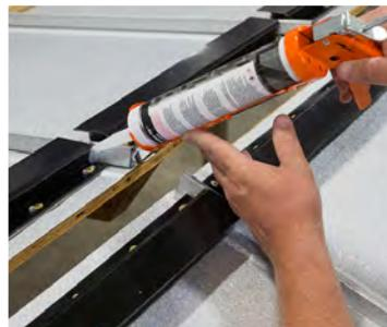
**STEP 4:** Apply sealant at the points where the SSV meets the panel ribs.
