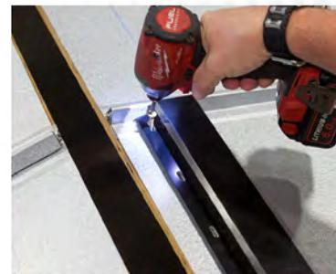
**STEP 3:** Secure the SSV using type 410 fasteners, ensuring at least one-half inch of penetration into the decking. Space the fasteners no more than three inches apart.
